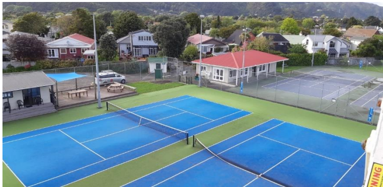
View from cherry picker replacing a light
