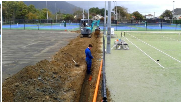
Cable ducting laid
